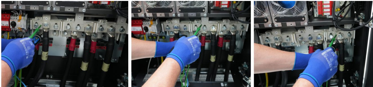
Abbildung 108: Isolationswiderstand DC+ / DC- am MCS-Dispenser
